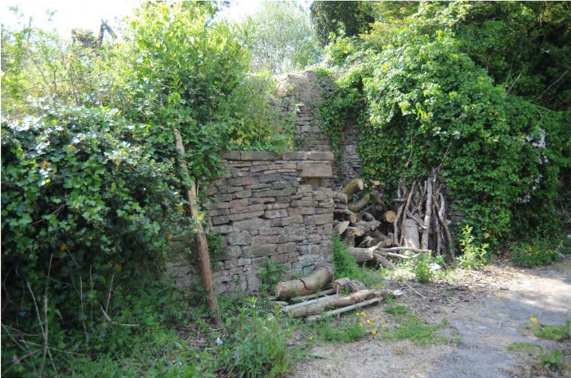
Pl.10: Rubblestone revetment wall on the drive to the north-west of the walled garden.
