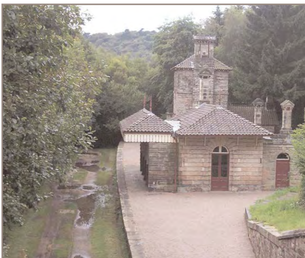
3.1 The Station buildings and track
