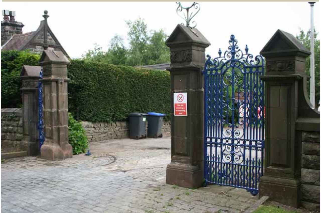
Drystone boundary wall in local pink gritstone, with gateposts ('stoops') and pyramidal caps. Right - remnants of the early wrought-iron spike railings and cast iron posts found around the damhead. Below - formal carved ashlar gatepiers at the entrance gateway to Horton Lodge, with bespoke wrought-iron gates, a very expensive addition
