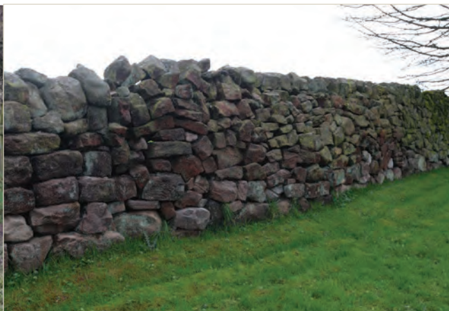
Above left - section of early, massive, boulder wall to the Rock House Farm croft. Above right - tall, dark red drystone wall to Brandon House Farm croft
