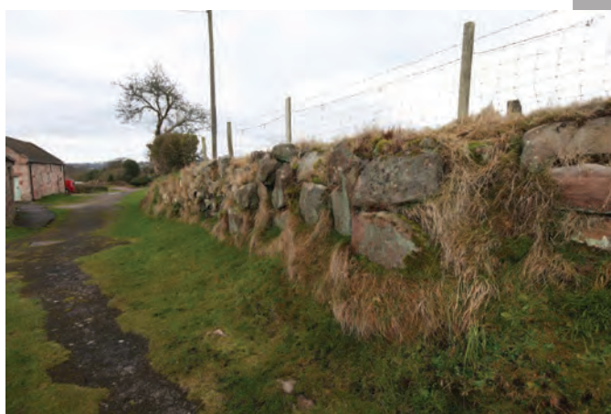
Massive boulder or 'orthostat' walls opposite Gate Farm
