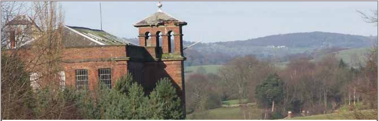
5.8 View from Overton Bank: Big Mill and beyond
