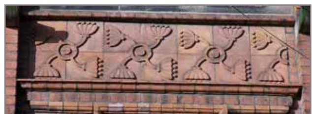
5.13 Queen Street: moulded brickwork
