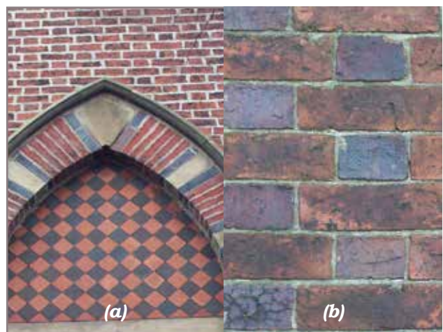
6.7 (a) Moulded brick (b) Flemish bond with dark headers.
