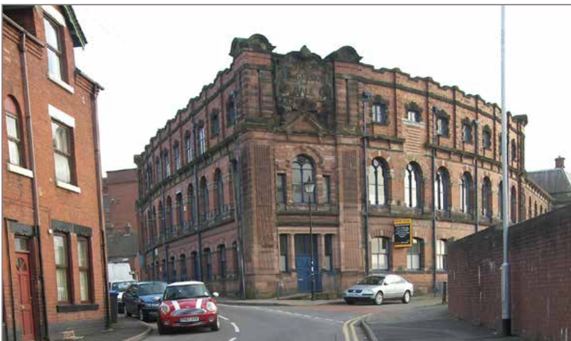
5.7 Cross Street Mill
