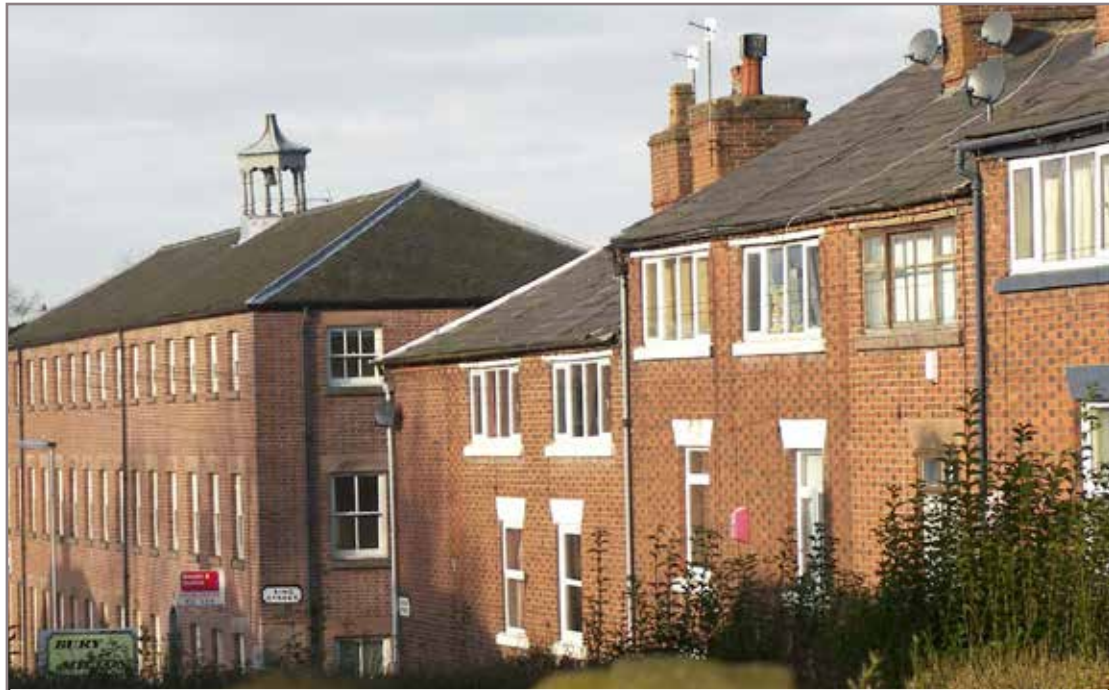
4.12 The earliest part of Albion Mill with the adjacent weaver's houses
