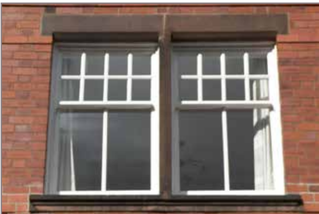
4.14 Sash windows with glazing characteristic of the period around 1900.
