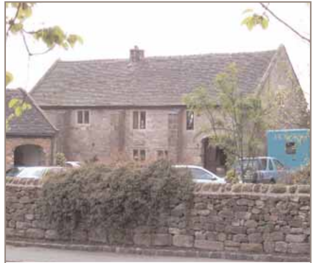
5.2 Bagnall Hall barn
