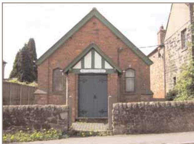
6.3 St Chad's Church Hall
