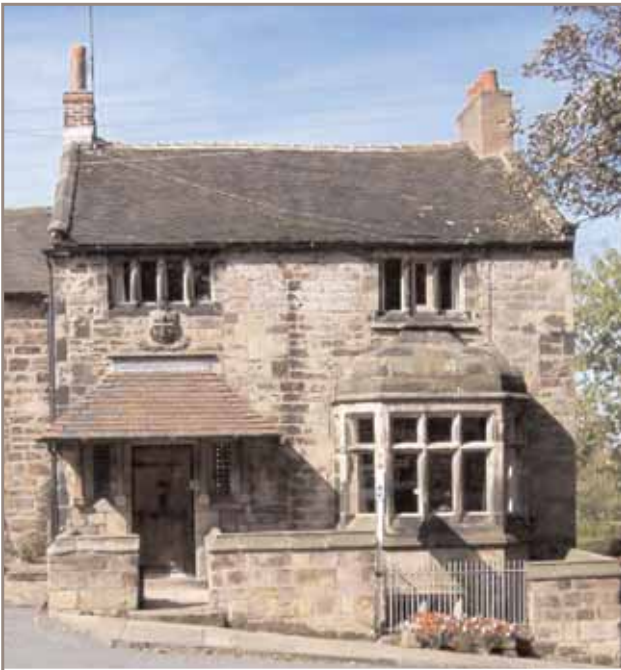
5.5 St. Chad's House
