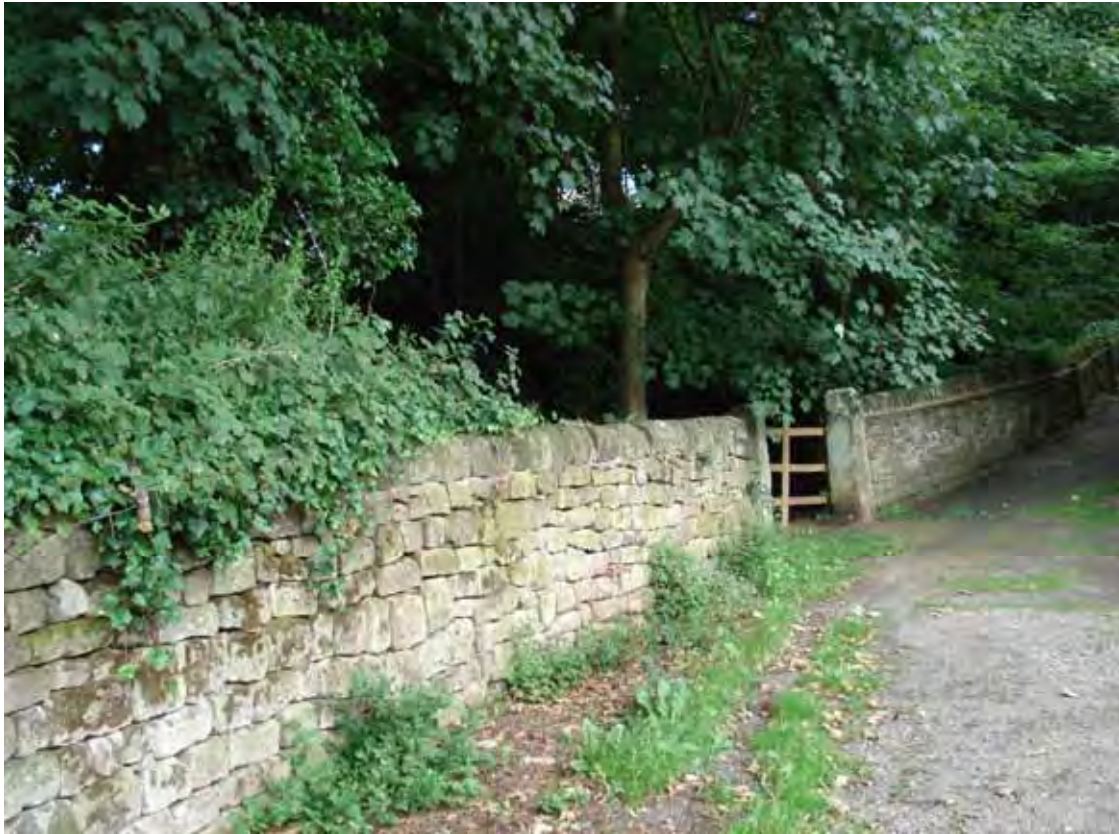
View to north from guesthouse carpark off New Road to the south of site
