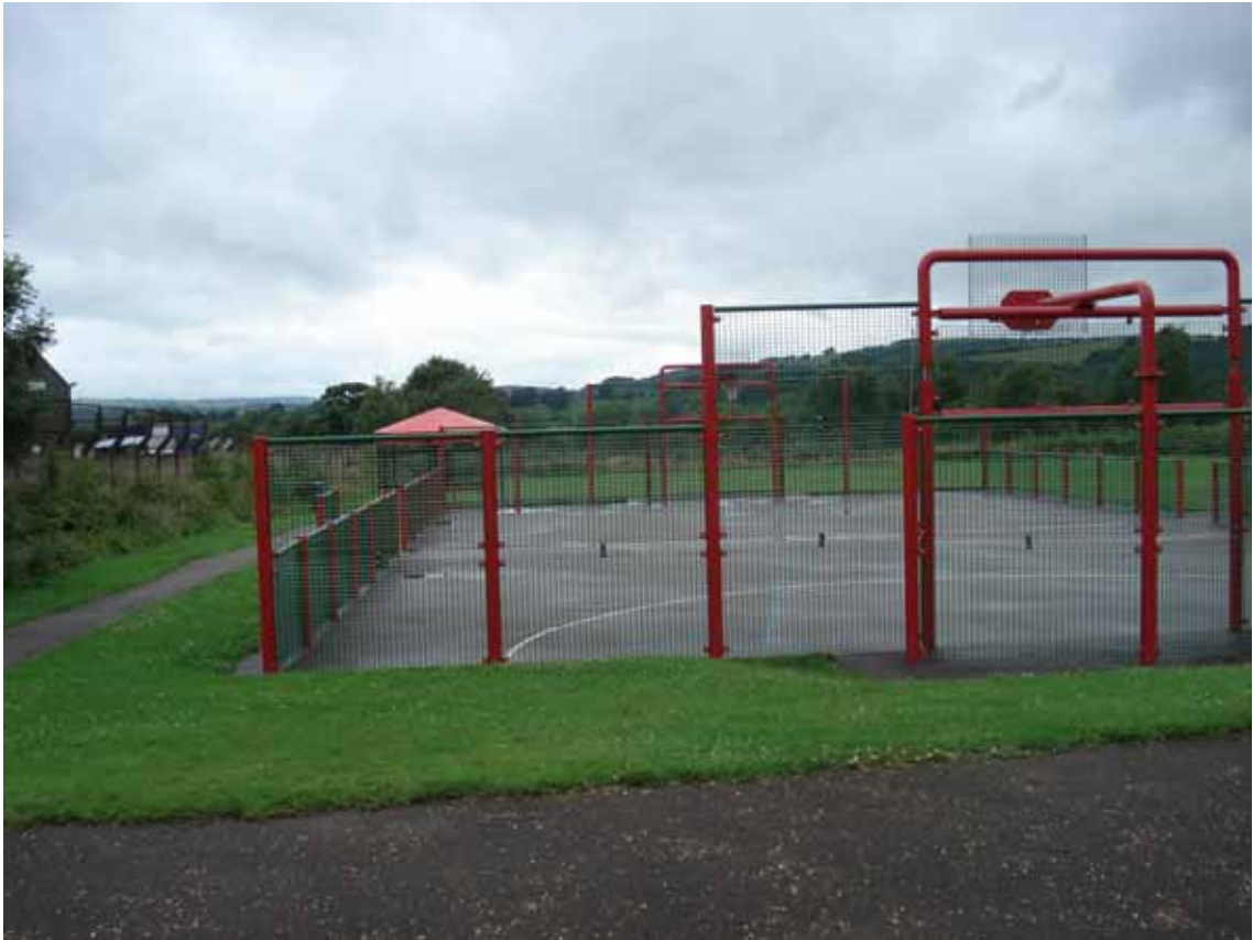
View to west from edge of site
