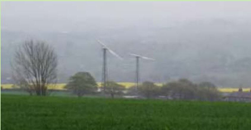
Two-bladed turbines with industrial-style lattice towers in a rural context (Source: LUC)
