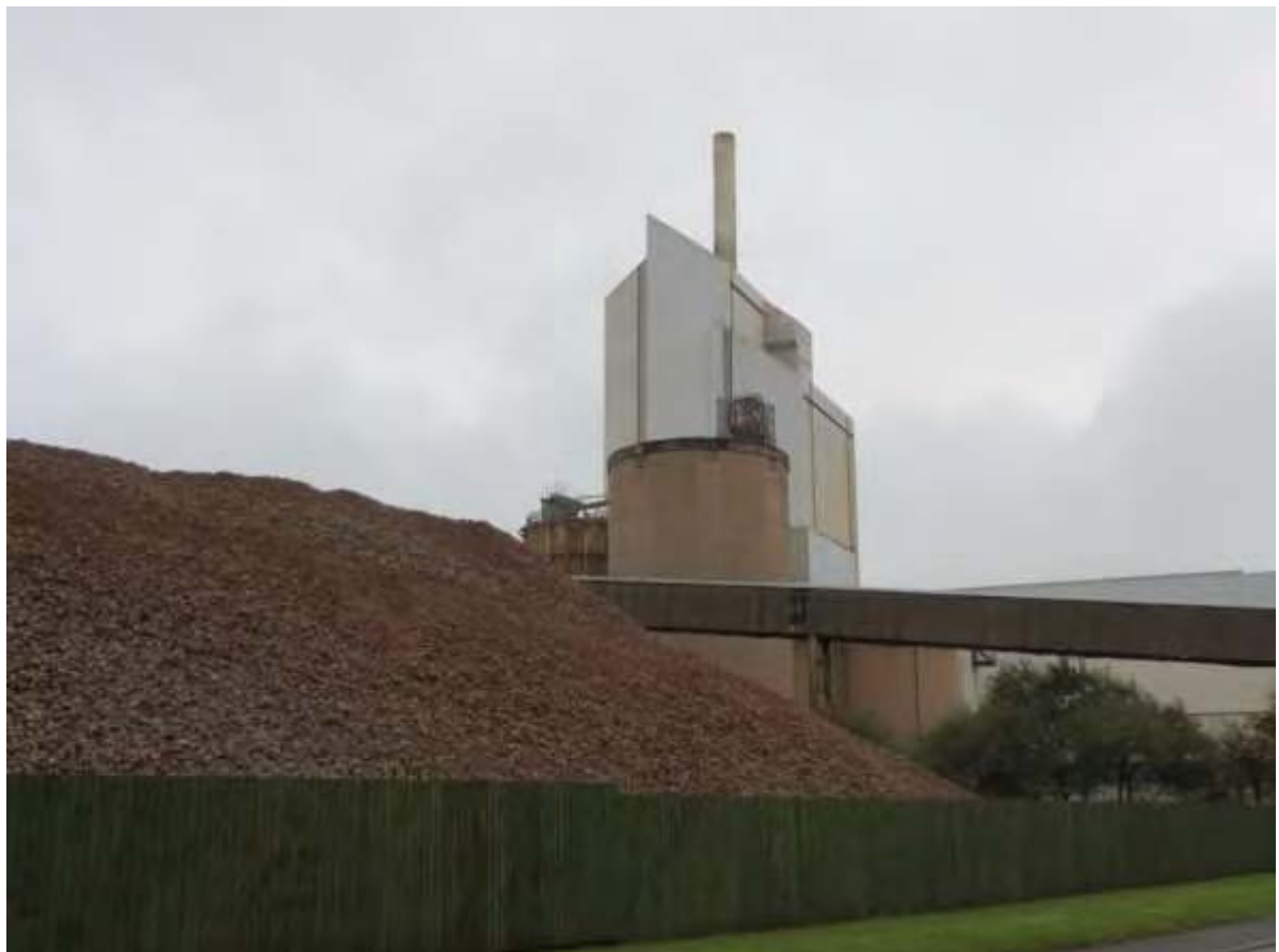
Figure 3.9: Caudon Low Quarry chimney (115m)
