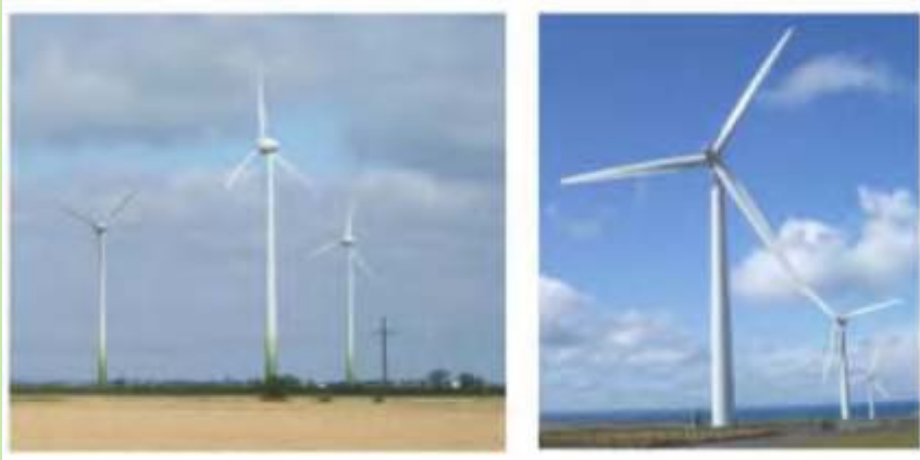
Examples of different rotor diameter to tower height proportions (SNH, 2014)
