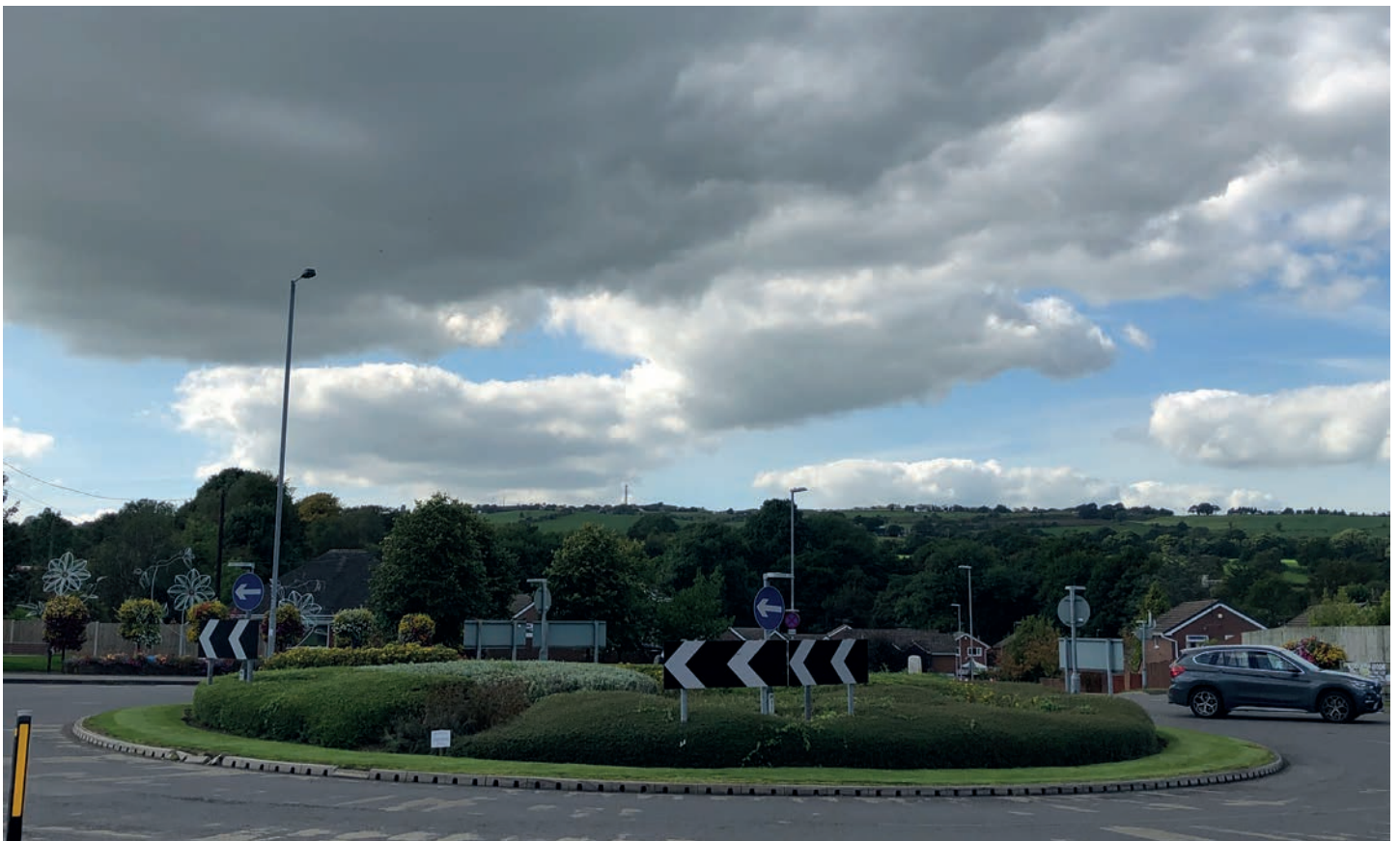
6. Wharf Road roundabout towards Mow Cop
