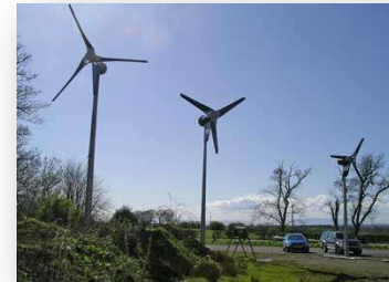
Wind Turbine Installation
