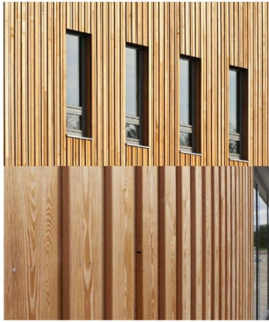
Board and Batten Stained Accoya Timber Cladding to over existing Brickwork
