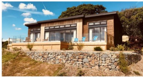
Typical Monopitch Timber (Vertical & Horizontal) Clad Lodge. Pale Grey Powder Coated Aluminium Frames. Galvanised Rainwater Goods. Pressed Metal roof. Timber Skirt and Deck Posts
