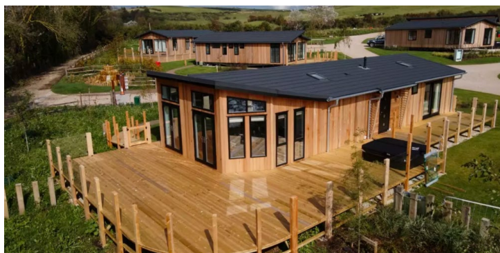
Figure 2: Lodge with raised and chamfered Lounge Roof
