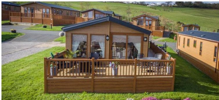
Figure 23: Example of lodges set out in straight rows with no soft landscaping included (not proposed under the Appeal Scheme)
