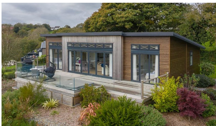
Figure 1: Mono Pitched Lodge Roof, with contrasting section of cladding
