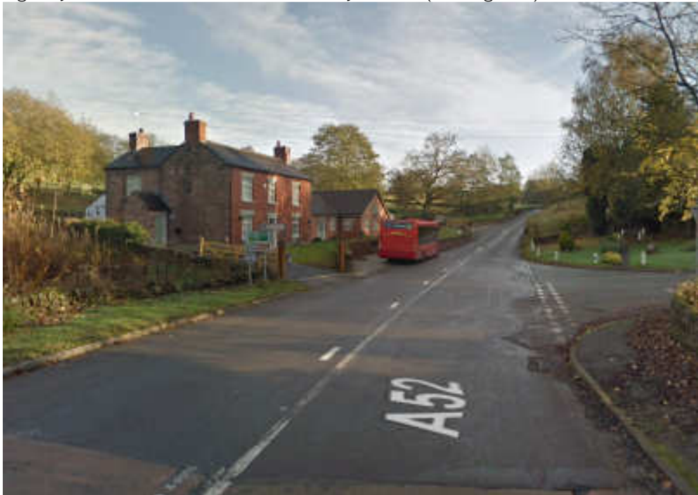
Figure JFRI. A52 / Whiston Eaves Lane Junction (looking east)
