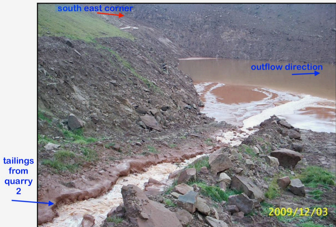
Plate 6.3 Quarry 3 – Tailings Inlet in north east corner
