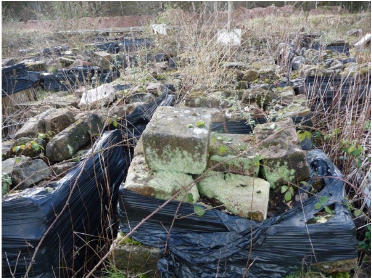
photograph S.2d Closer view showing brambles and bushes growing in between the stone piles.
