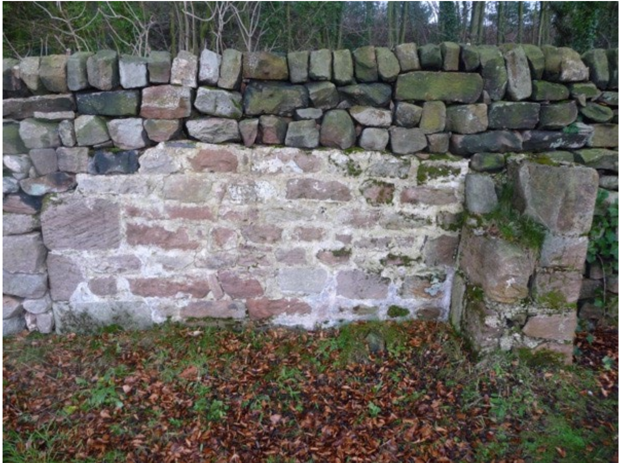
photograph A.4c Shows a lime mortar bonded section of an interior wall of the building within the matrix of the modern roadside wall as seen from the western or quarry side.
