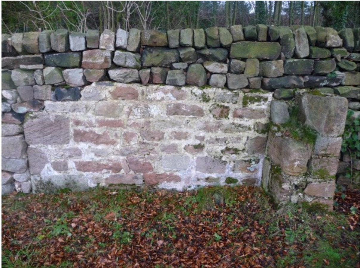
photograph A.4c Shows a lime mortar bonded section of an interior wall of the building within the matrix of the modern roadside wall as seen from the western or quarry side.
