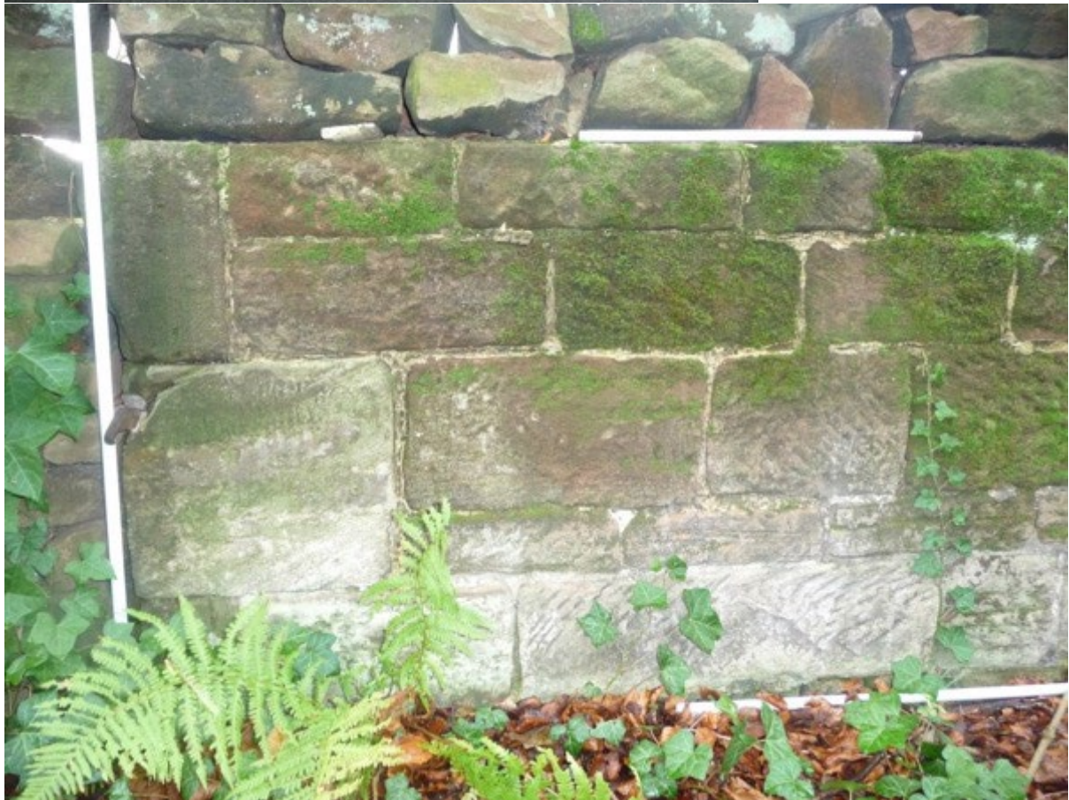
photograph A.4b Photograph A.4b shows a close up of a section of the original stable block building with finely tooled, dressed ashlar courses bonded in their original positions
