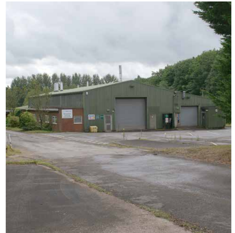
Above: View of retained building within Quarry (to be the ‘activity building’)
