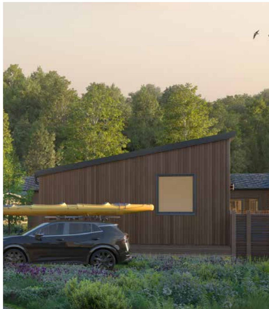
Above: From the CGIs, a flank view of one of the lodges illustrating a mono pitch roof, integrated skirt base and flank timber elevation, defined enclosed eaves. One design detail of the lodges
