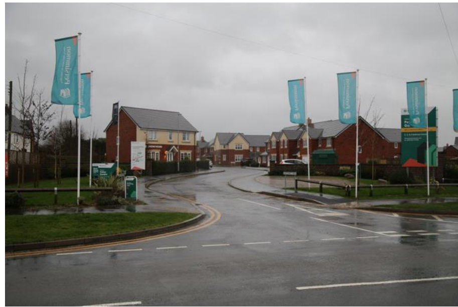
Plate 28 – Potters Gardens has been built out by Persimmon Homes on the allocated site CH001 to the south of the Appeal Site by 340m.
