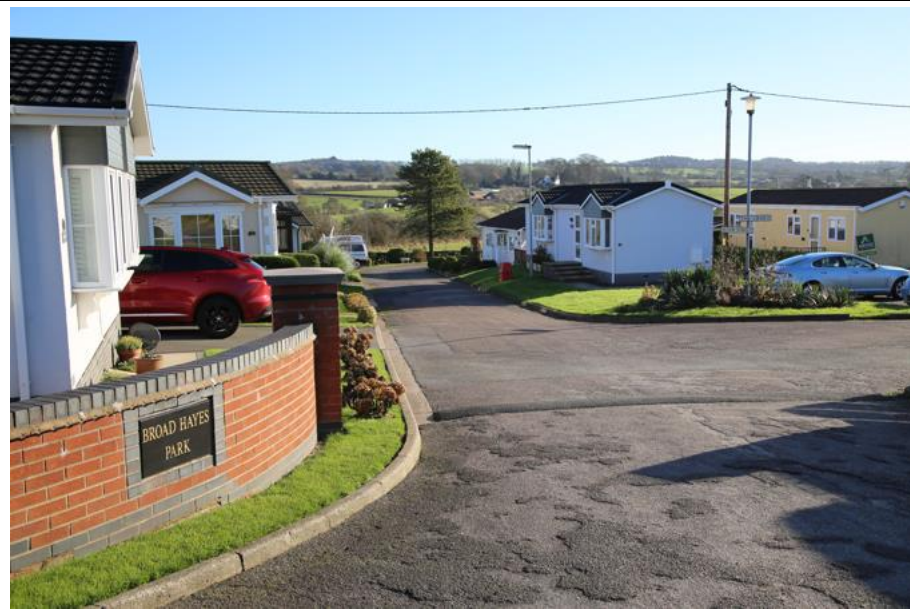
Plate 11 – Broad Hays Park sits to the south of Hammersley Hayes Road and consists of single storey park homes. Allocated site CHI32 is set beyond park.
