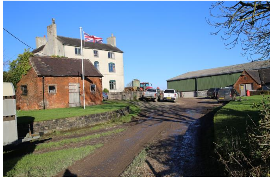
Plate 13 – Broad Haye Farm with the Grade II Listed, white painted three storey farm house set within a collection of modern and older farm buildings.
